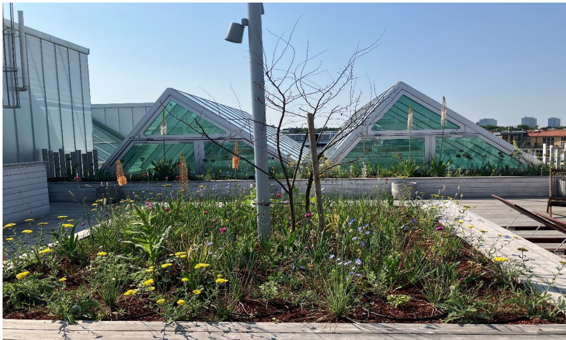
Photo 10: Plants on the roof terrace
